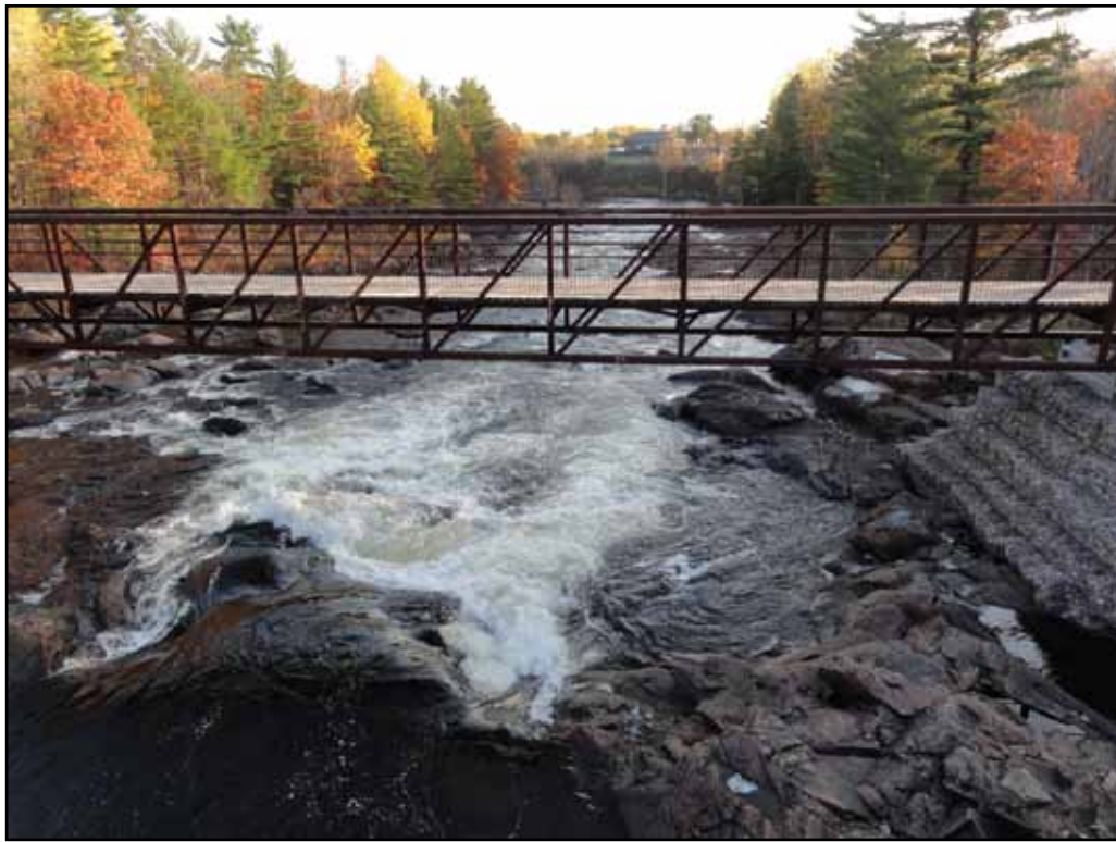
Photo 14. Big Eddy rapids, looking downstream from the railway bridge.
