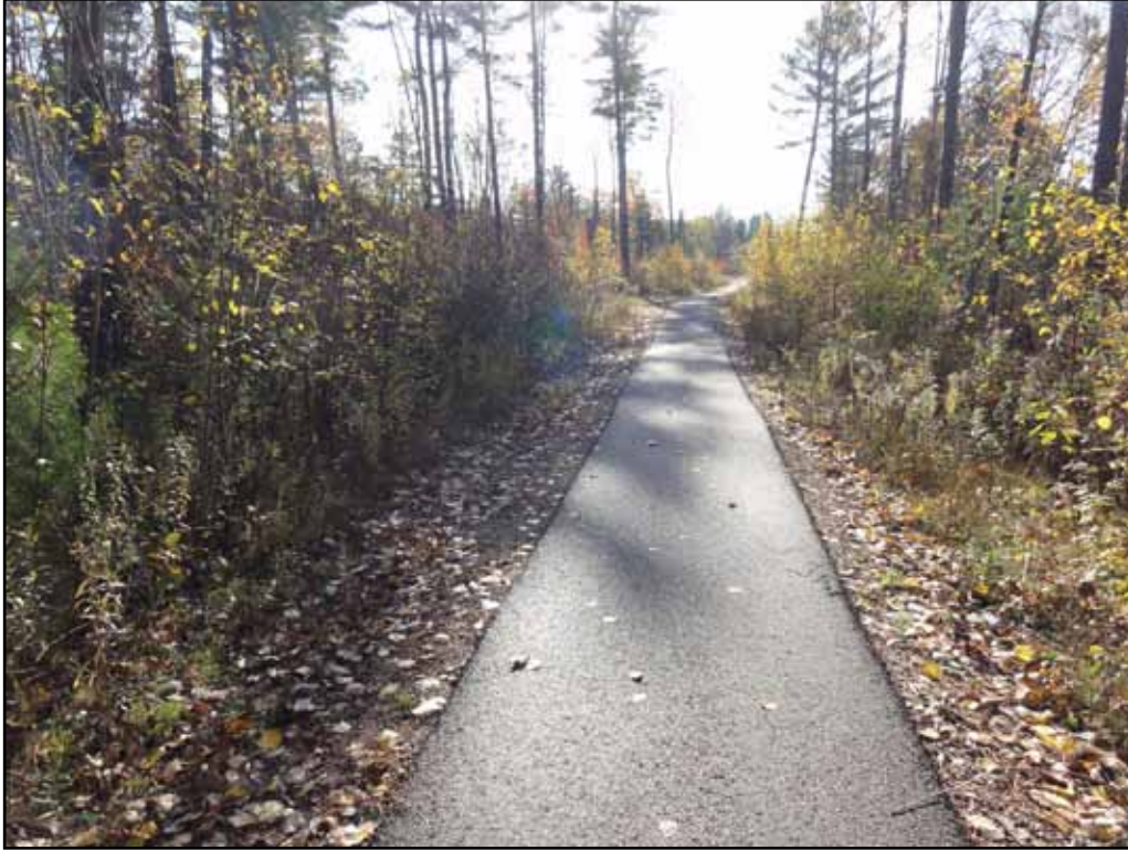
Photo 23. Asphalt trail in the park in Area C, north shore of Petawawa River.
