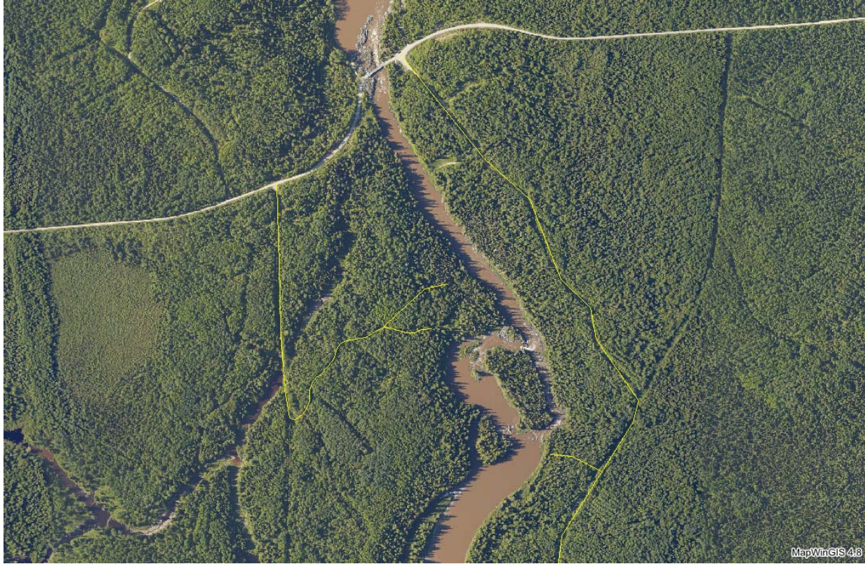
Figure 4. Imagery showing access to the East and West side of the generator
