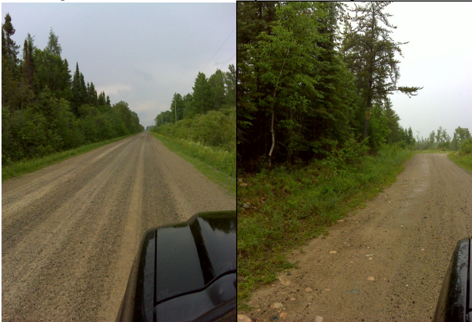
Figure 6. Primary and Secondary roads sections along the Ice Chest Road.
