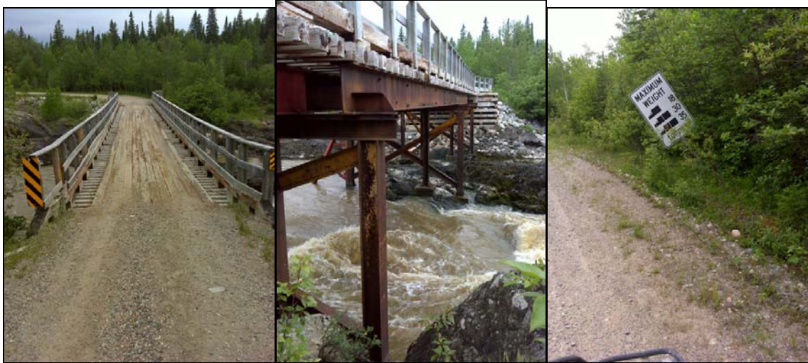
Figure 2. Bridge crossing the Frederick House River.
