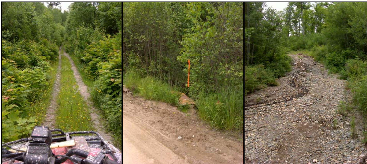
Figure 1. Examples of areas requiring upgrade or repair along existing Eacom roads.
